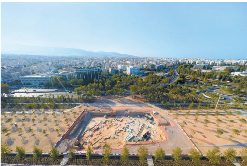
Aerial photograph of the Esplanada excavation site at SNFCC.
